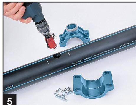
6. Assemble the saddle according to the marked lines; to keep the hole in axis with the branch direction it can help to use a pin, such as the drill used to make the hole.
